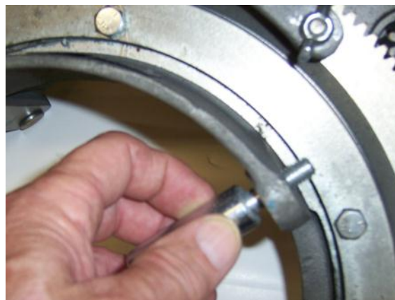
Picture 2 – Installation of Spacer Bolt
